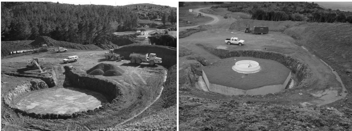
Figure 1: Stages of foundation construction
