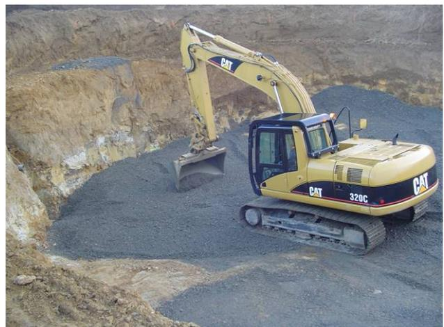
**Figure 7:** Backfilling of undercut at Site 34.
