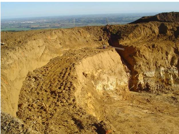
**Figure 6:** Site 34 excavation and undercut concrete pad. Founding level is approximately at the PVC pipe level.
