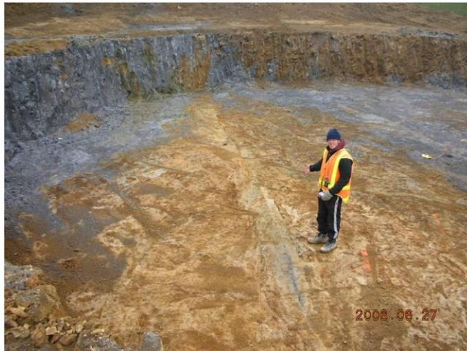
**Figure 5:** Clay filled lineament through second foundation excavation at site 9.
