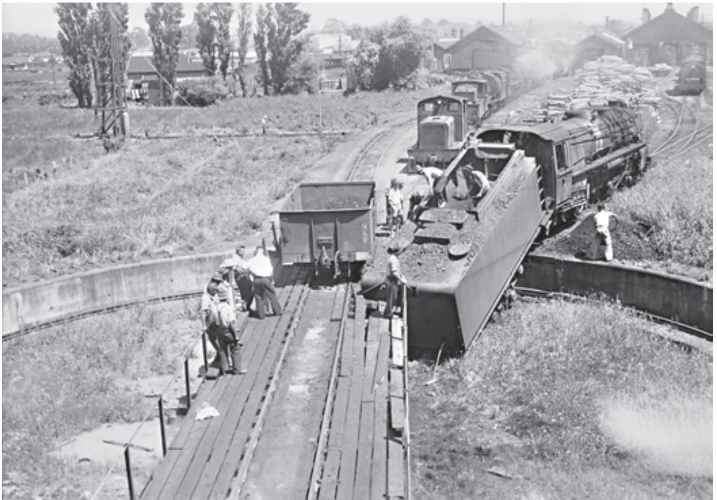
1947 CHRISTMAS DAY MORNING MISHAP SHOWING THE TENDER OF K 908 IN THE TURNTABLE PIT. THE DRILLING RIG AT LEFT WAS BEING USED TO ESTABLISH FOUNDATIONS FOR THE INSTALLATION OF FUEL OIL STORAGE TANKS - JAT TERRY
